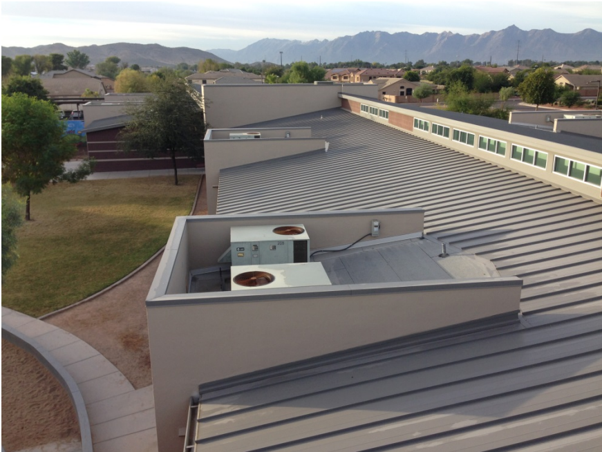
Typical mechanical enclosures at metal roof
