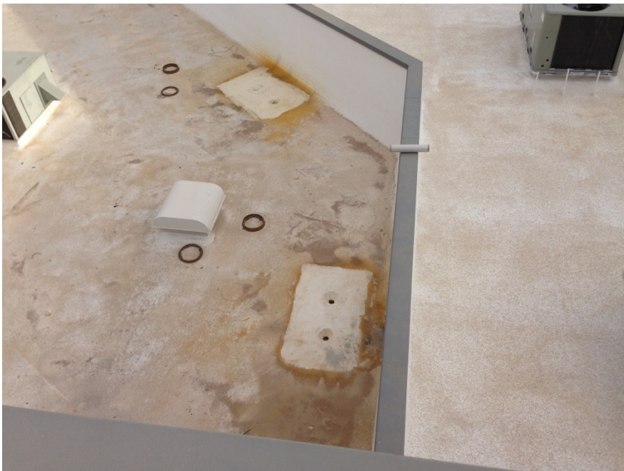
Repaired roof drains adjacent to addition
