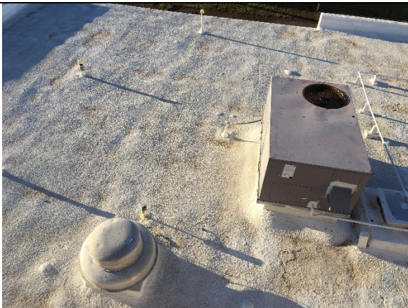
Building C blistering lower roof
