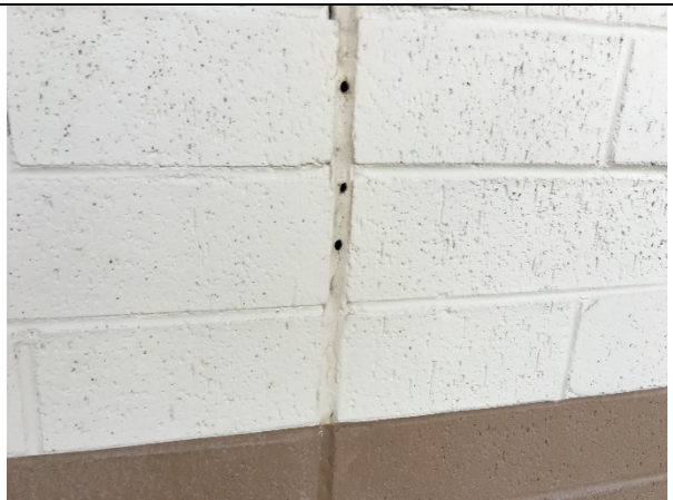
Building A failing caulk joint
