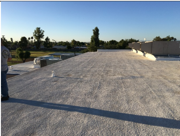
Building C typical overview – BUR lines telegraphing through the foam
