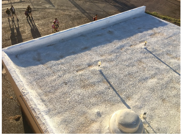
Building C blistering lower roof
