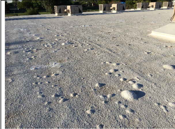
Building A typical blistering
