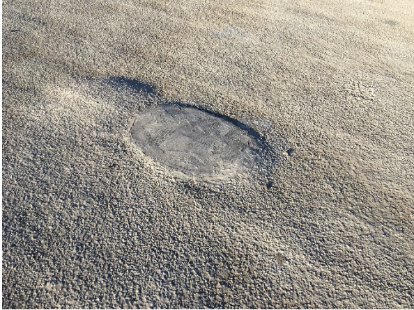
Building C improper blister repair
