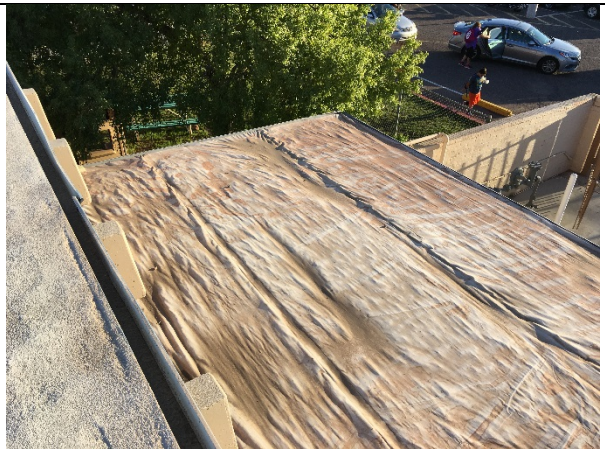
Building C – single ply failure at lower roof
