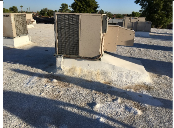
Building A blistering and HVAC curb
