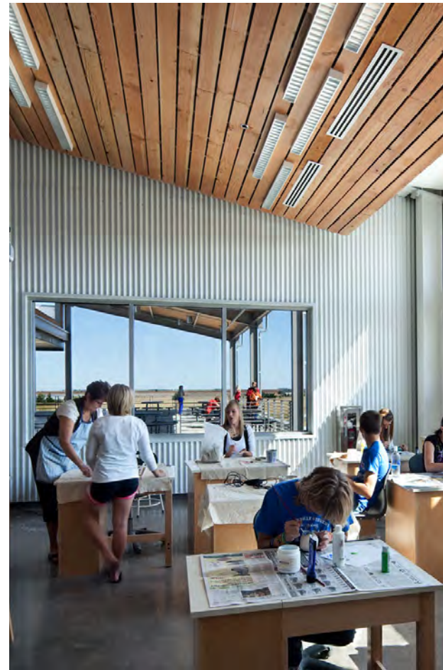
Low operable windows for natural ventilation provide the teacher control over the classroom environment. (Kiowa County Schools, Greensburg, KS; BNIM Architects)
