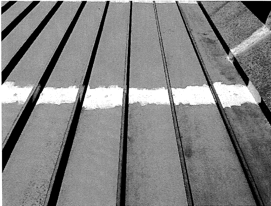
Screw holes sealed with elastomeric
