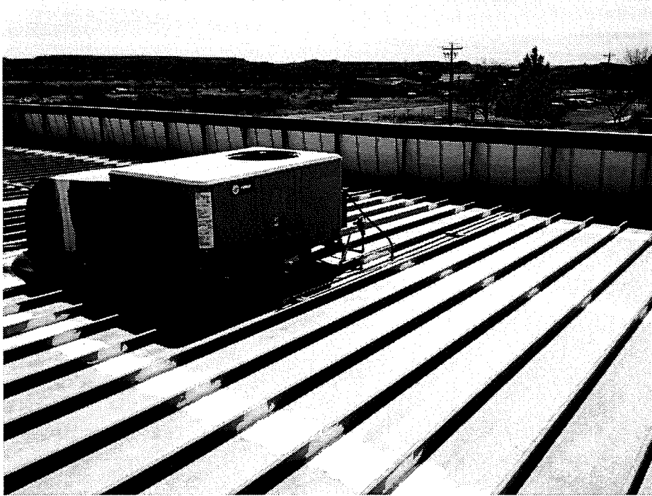
Roof top units sitting on racks with side draft duct work
