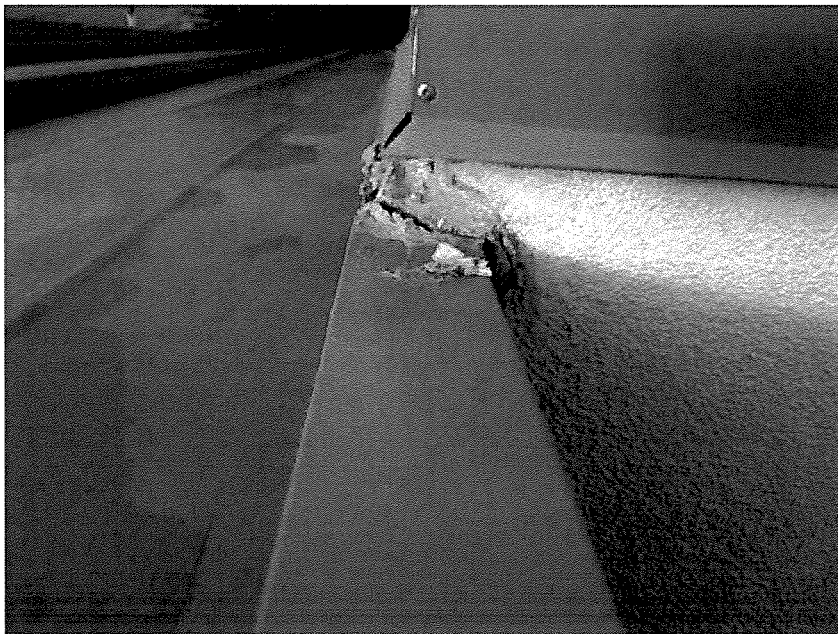
Perimeter sealant voids at metal roofing
