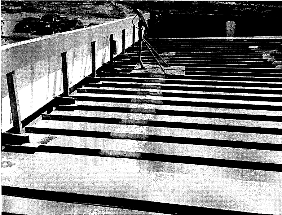
Mansard equipment screen with integral gutter
