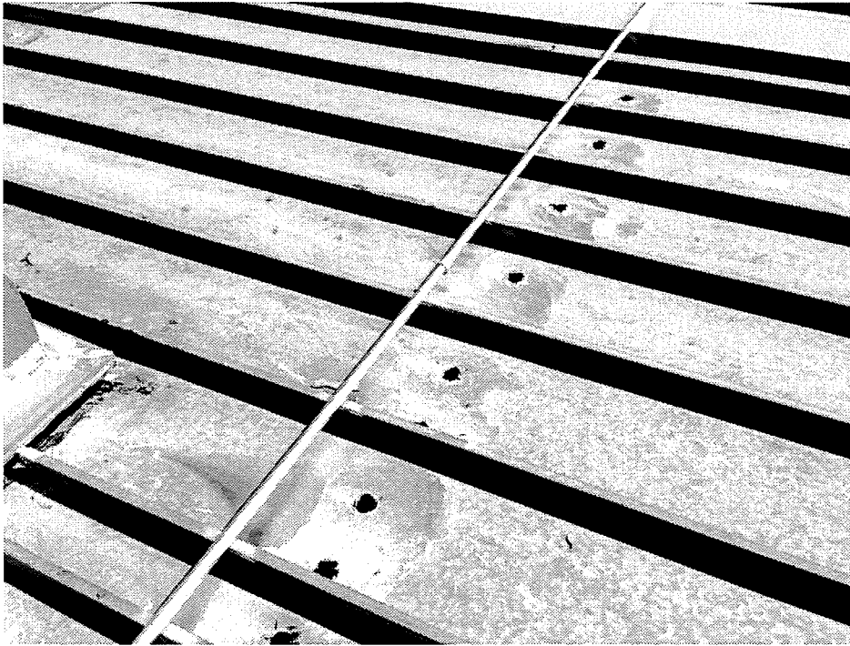
Note roof panels attached using Tek screws
