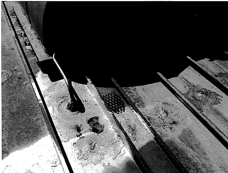
Improper conduit penetrations and screw holes sealed with roofing cement
